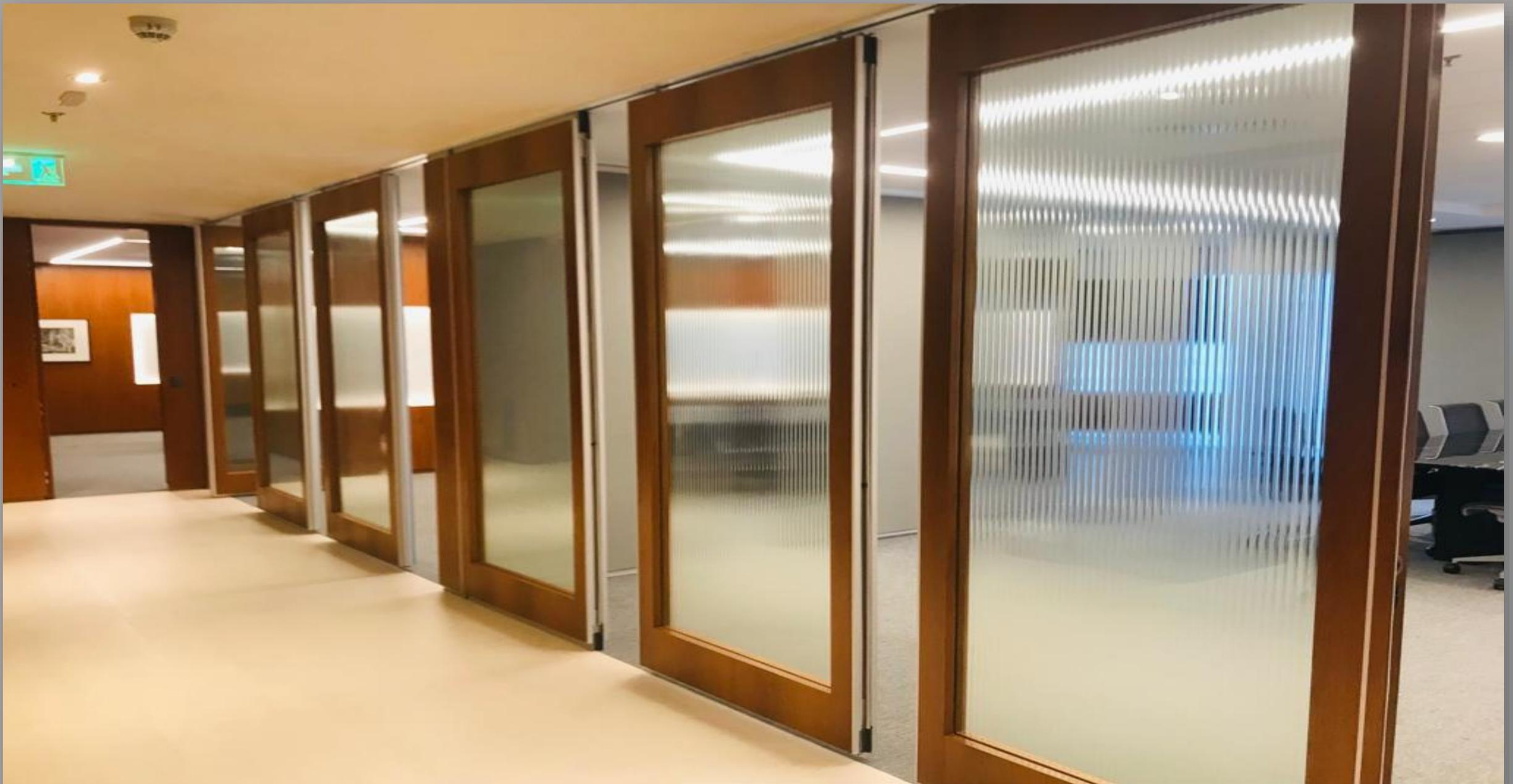
**Modelo Standard – Rev. Painel especial c/ vidro canelado**
